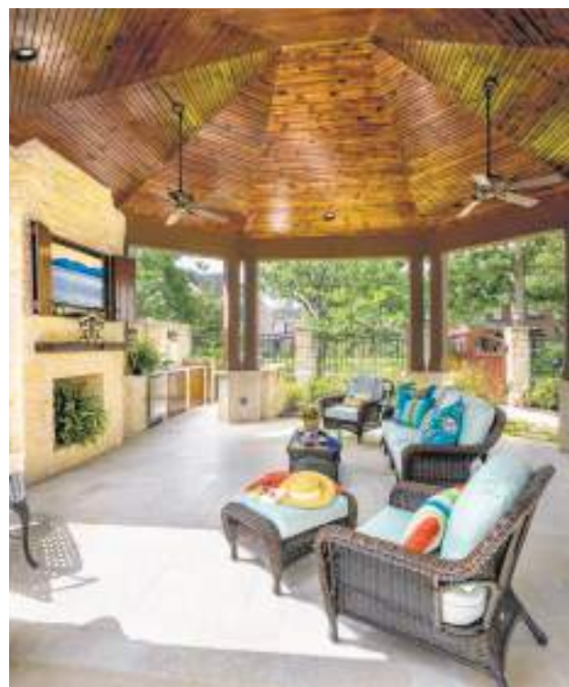
Custom-milled cedar columns hold up the eight-sided vaulted ceiling that's covered underneath with stained pine.
